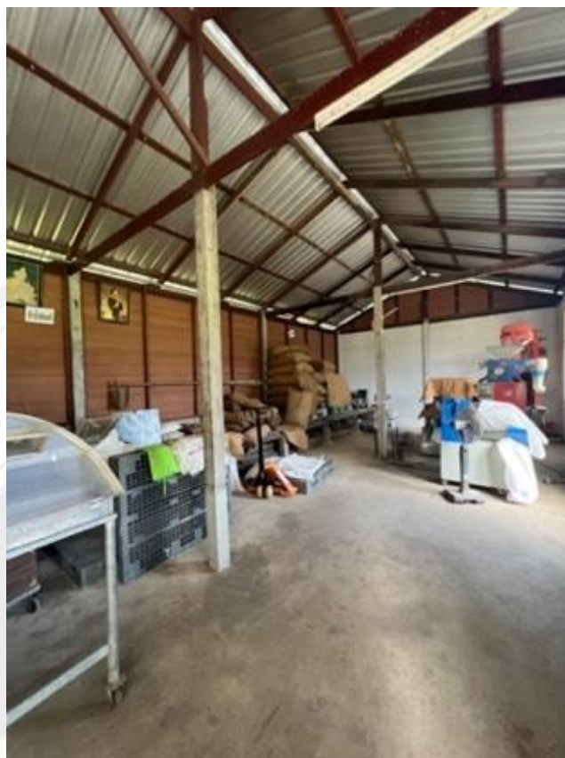
Figure 4.19 Interior of Rice Mill with Budget Support from Provincial Energy Office-Nakhon Pathom, Ministry of Energy
