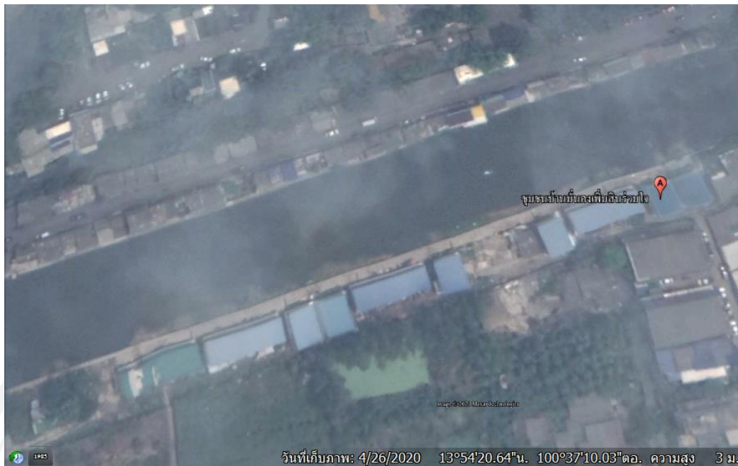
Figure 4.4 Phermisin Ruamjai Community after the Waterside Housing Development Project.
