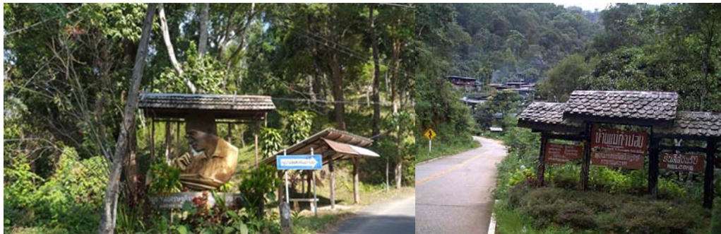
Figure 4.1 Road and Entrance to Ban Mae Kampong Homestay
