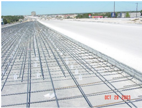
Reinforced concrete pavement (Rd_1)
