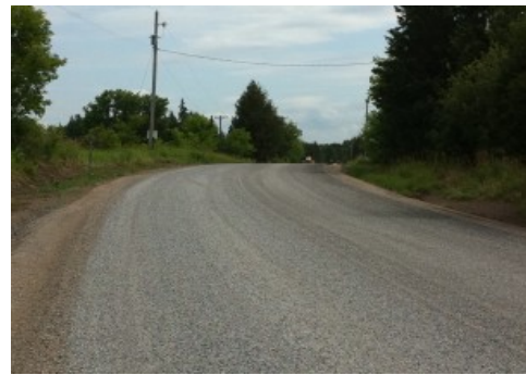
Double surface treatment (Rd_2)
