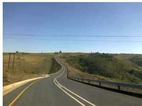
Cape seal pavement (Rd_4)
