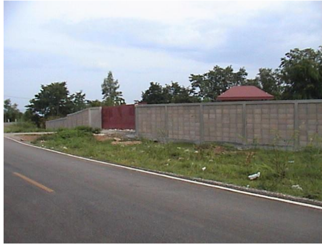
Figure F4 Surrounding Area of Landfill Pit in Koh Kha
