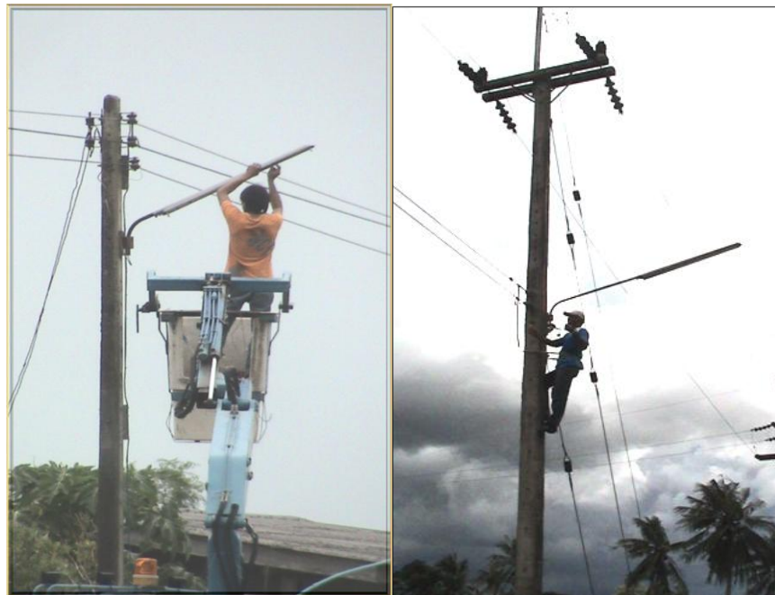
Figure D8 Electricity Fixing on Site
