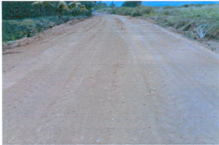
Figure D7 Larterial Road in Tambon Ta Sit
