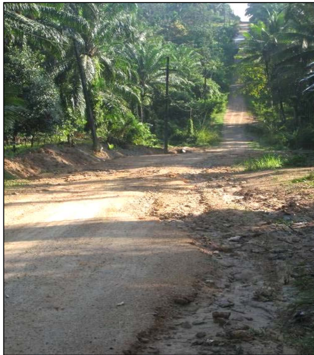
Figure 5.15 Condition of Street One Month after Reconstruction
